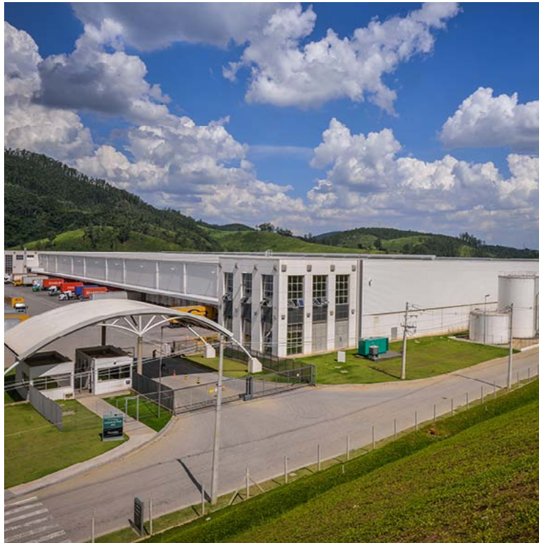
Prologis CCP Cajamar Industrial Park, Sao Paulo, Brazil
