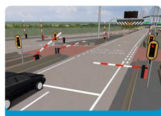
Barriers will be used in conjunction with traffic signals to stop vehicles and enforce crossing restrictions when required.
