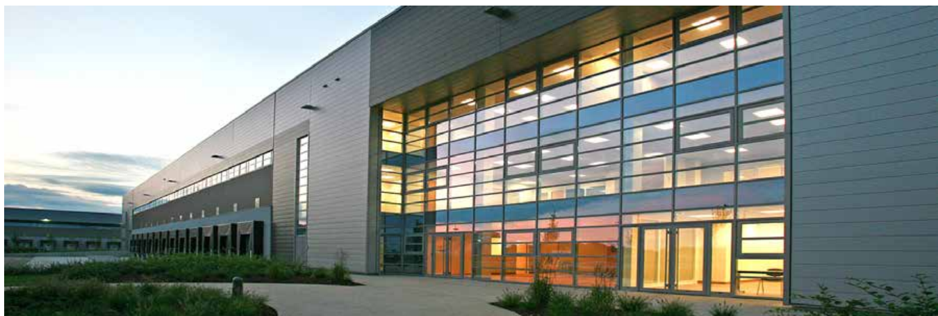
Prologis Park Chanteloup, Moissy-Cramayel, France.
